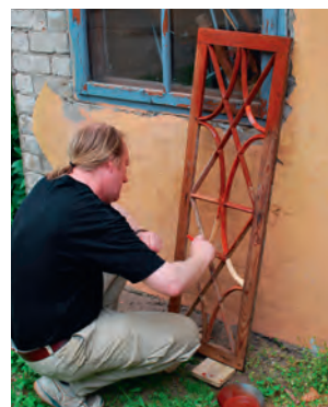
Overlysvindu i Jelgava gate 9
