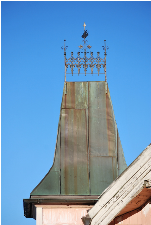
Skivetekking, kobber. Tårnhuset, Drøbak
