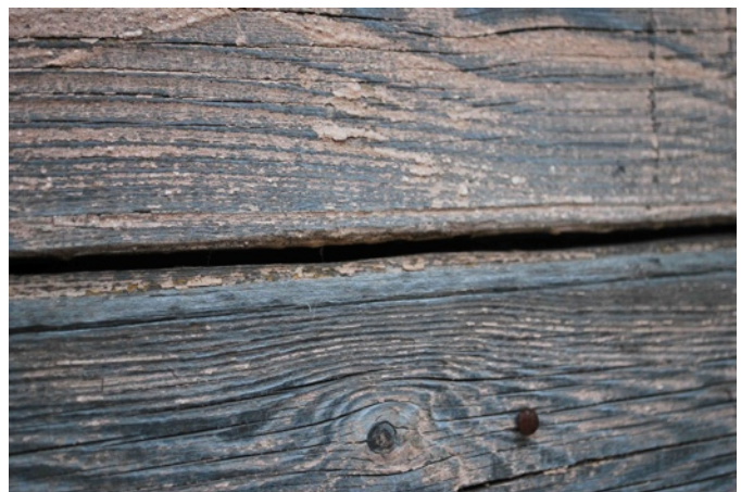
17. Baznica iela 7, Panels/boards. Baznica gate 7, Panel/ kledning.
