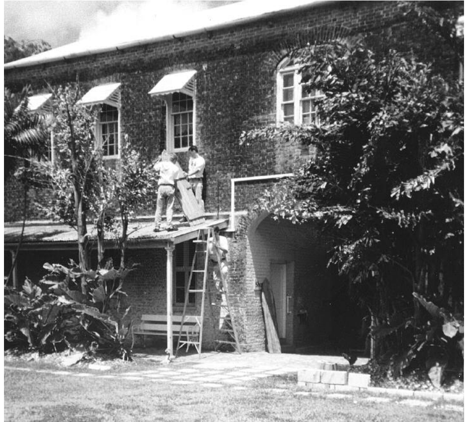
Figure 7 Buildings and maintenance staff of the Barbados Museum and Historical Society installing shutters on the museum's windows to protect against an advancing hurricane. Courtesy of the Barbados Museum and Historical Society. Photo: Alissandra Cummins.
